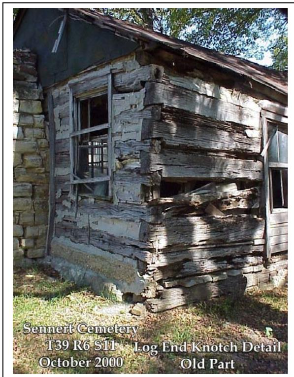
The picture on the left shows the detail of how the logs were notched on the original part of the log cabin.
