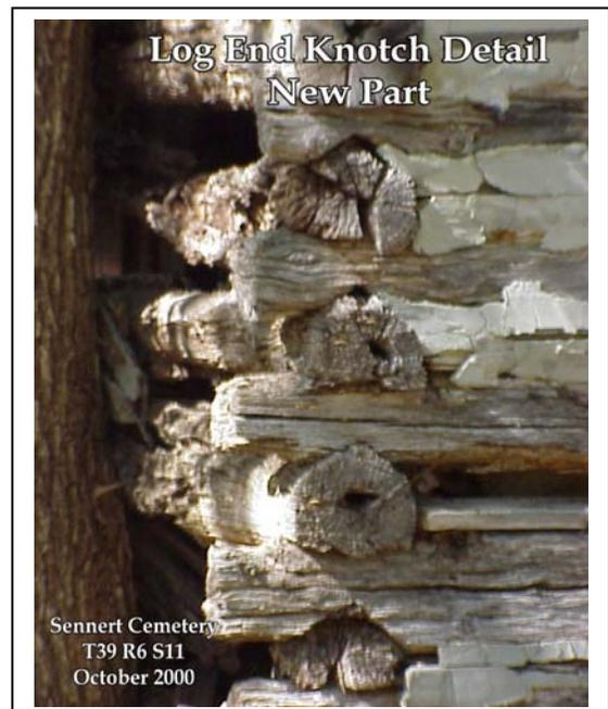
Picture at right shows notch detail on the newer addition.
