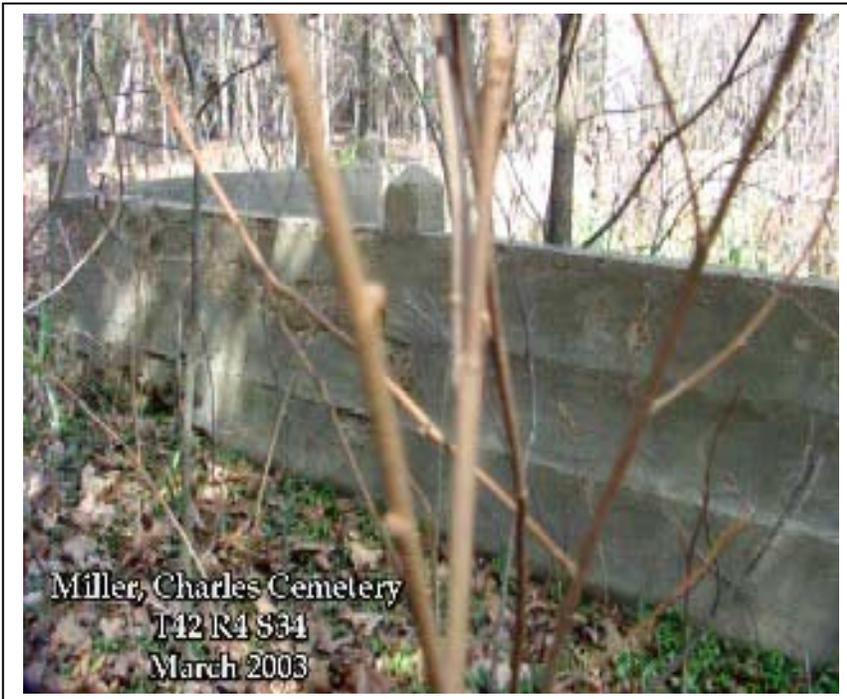
The photograph at left shows the concrete wall surrounding this cemetery. The concrete is starting to crumble in places as can be seen in the photo.
